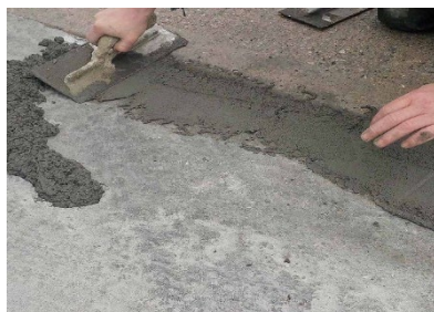
Repair of surface imperfections using cementitious repair mortar
